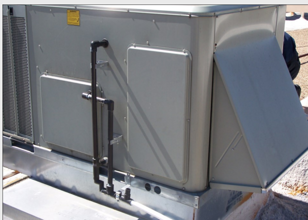
Figure 4. Typical installation of a CostGard™ Condensate Drain Seal System
