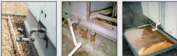
Figure 1. Typical trapped systems that meet industry codes
